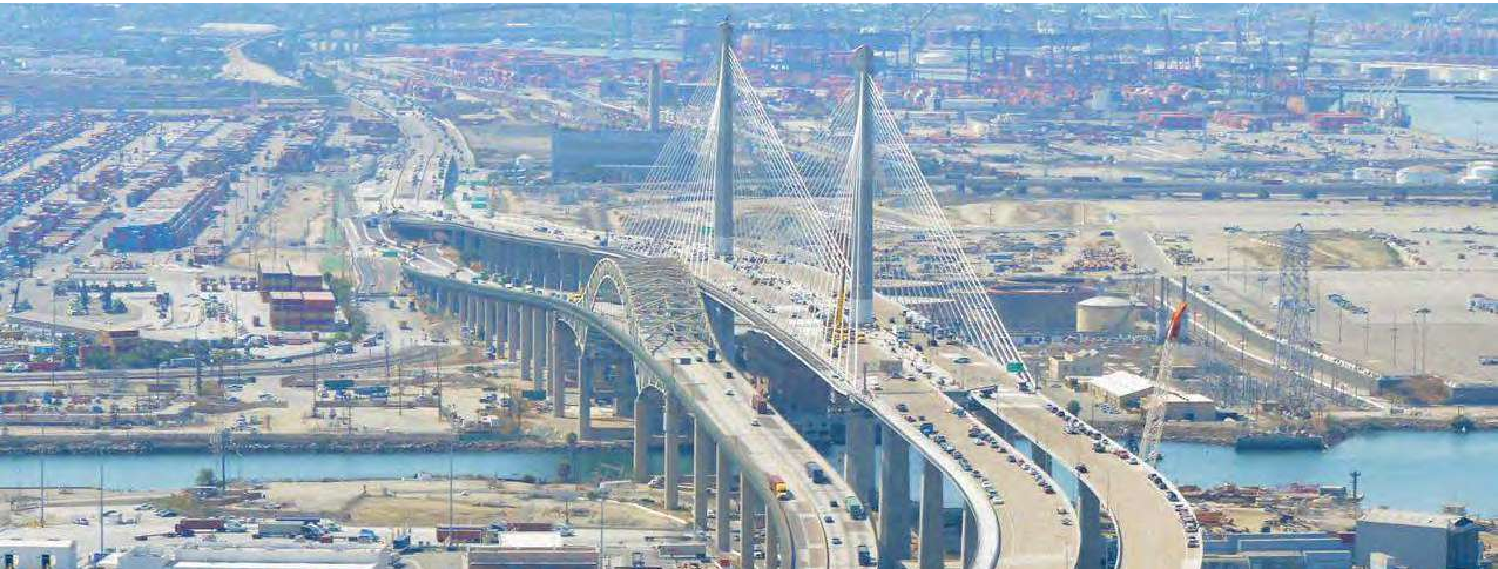
Gerald Desmond Bridge, USA
