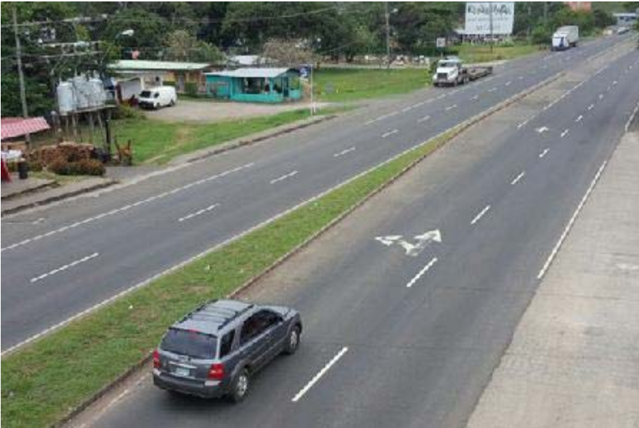
FCC wins tender to expand sections I and II of the Inter-American Highway (Panama)
