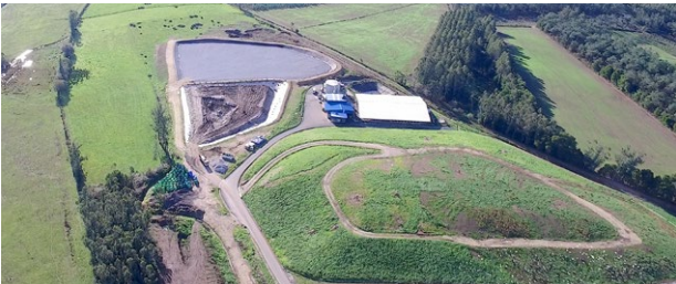
Degasification and restoration, Barbanza landfill.
