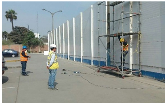
View of the panels from inside the Jorge Voto Bernales Hospital.
