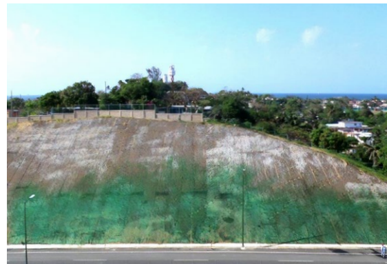
Hydroseeding on the sides of the embankment.
