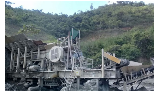
Dust mitigation systems using pipes and pumps.
