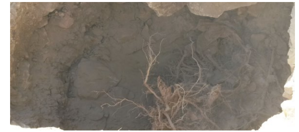
Removal of stumps, roots and surrounding soil.
