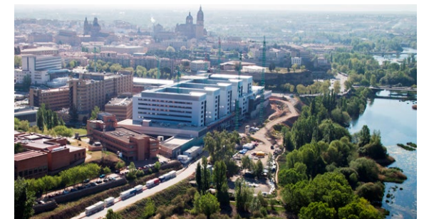
Area before and after the project.
