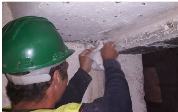
Works to exclude bats.
