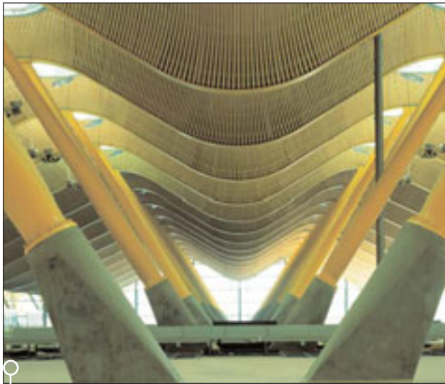
ON THE TOP, PRESIDENT JOSÉ LUIS RODRÍGUEZ ZAPATERO, the President of the Madrid Autonomous Region, Esperanza Aguirre, the Minister of Development, Magdalena Álvarez, and Madrid's mayor, Alberto Ruiz-Gallardón, at the official inauguration of Terminal 4. Below, detail of the new airport building.
