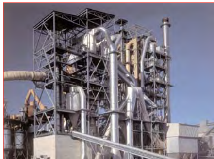
Detail of the factory.
