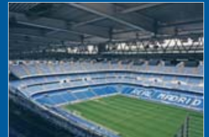
From top to bottom: some of the projects of similar characteristics built by FCC in other cities: Allianz Arena in Munich; the new Real Murcia soccer field known as Nueva Condomina; and the Santiago Bernabéu soccer stadium in Madrid.
