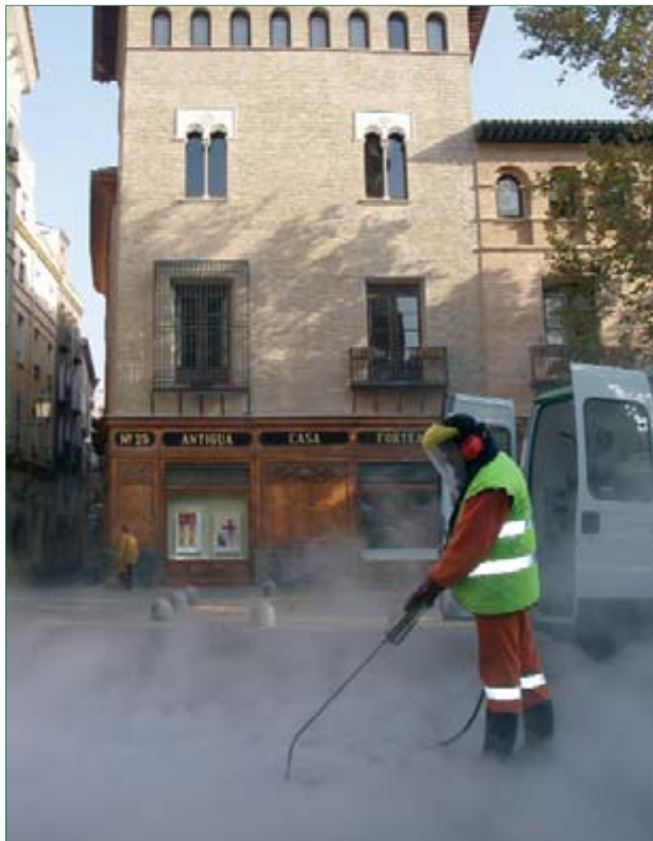
Gum and stain removal in sidewalks.
