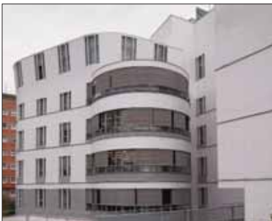
Above, the Esther Koplowitz Biomedical Research Center (CIBEK) and La Casa Nostra Fort Pienc for the elderly in need (Barcelona).
