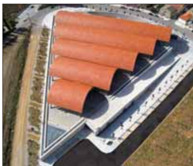
The facilities are situated at the foot of a hill crowned by a medieval castle.
