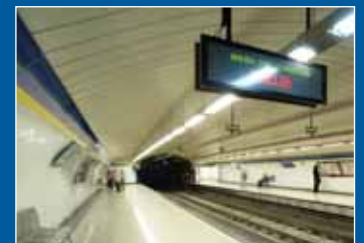
Above, the Guadarrama Tunnel and, above these lines, the platform at Line 3 of the Madrid subway system.
