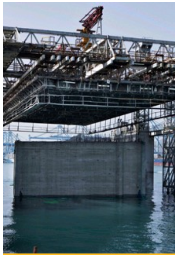
Coffer ready for launching
