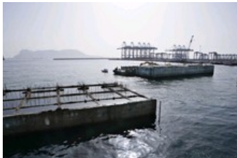
Manufactured coffer for pier construction
