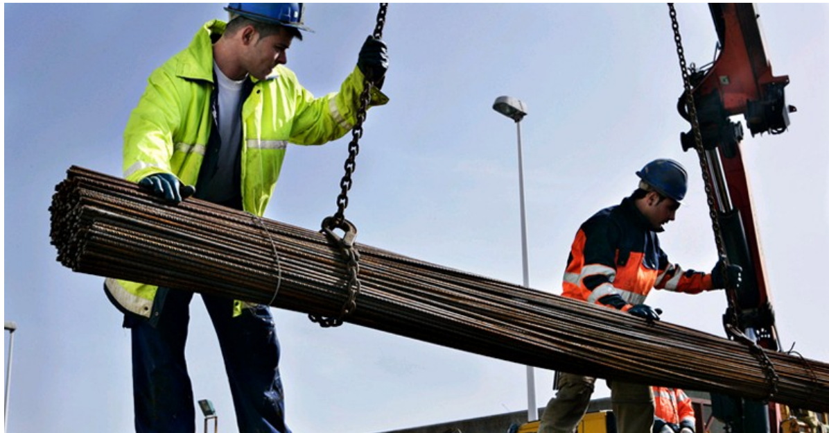
Workers at the steel framework park
