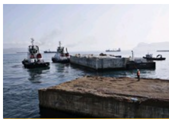
Transferring the coffer to its definitive location
